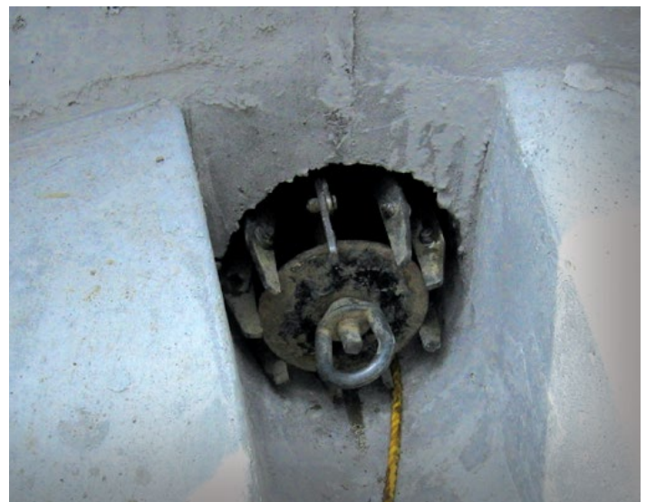
Mandrel test starting at a Maintenance Hole
