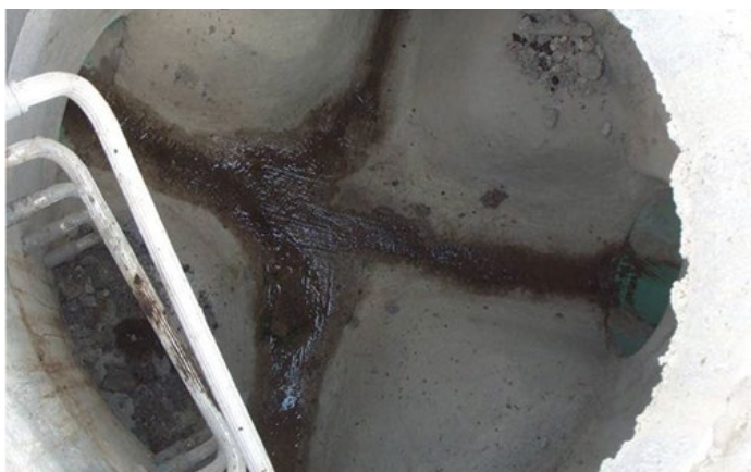
Figure 1 - Typical Field Benching
