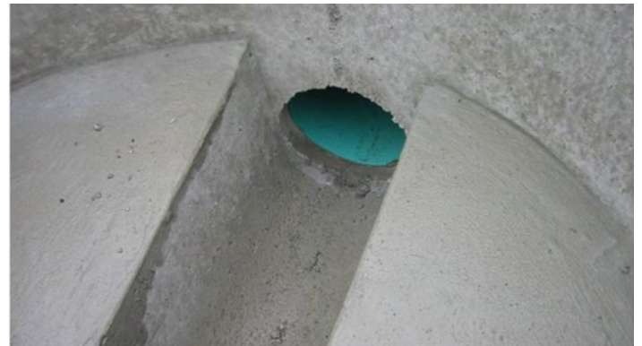
Figure 2 - High Quality Precast Benching
