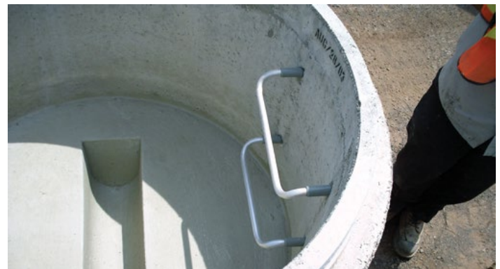
Figure 4 - Factory Produced Benchng
