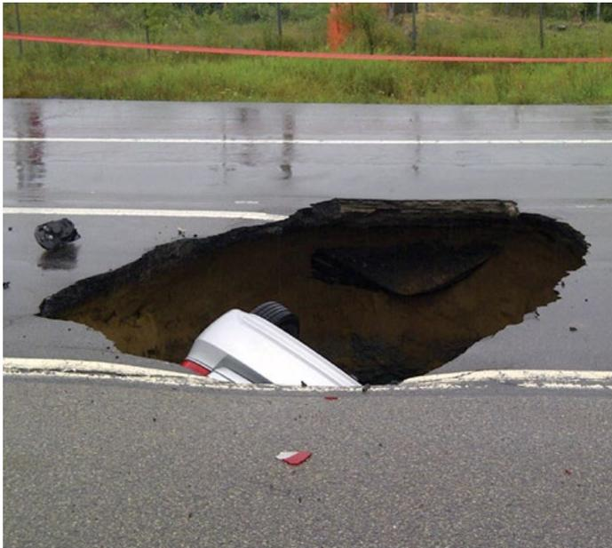
*Car falls into Highway 174 sinkhole after steel culvert collapses underneath
