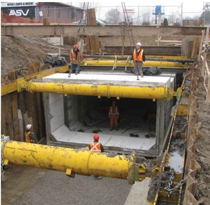
Reinforced Box Culvert for a storm sewer under a busy street
