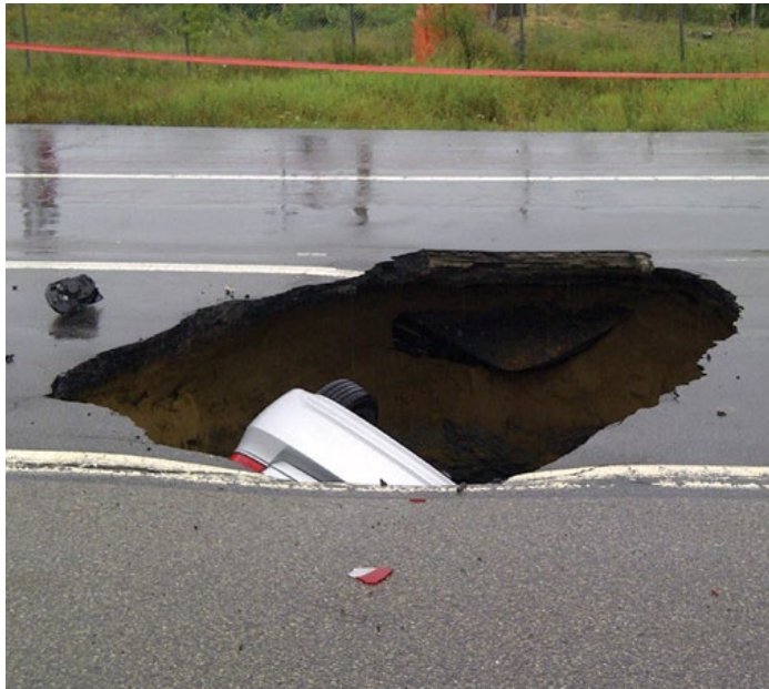
Car falls into Highway 174 sinkhole after steel culvert collapses underneath Courtesy: Ottawa Fire Services
