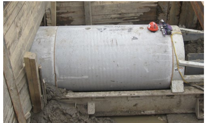
Jacking concrete pipe under Manitoba Highway
