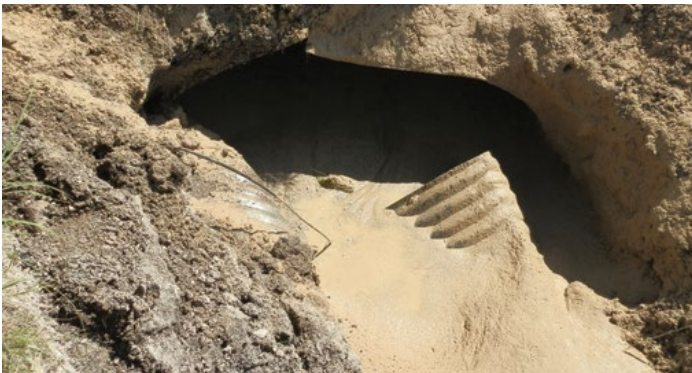
Decommissioned CSP culvert being filled with concrete
