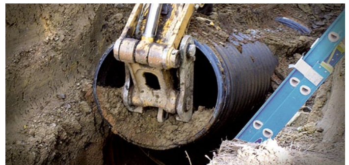
Reinforced Concrete Pipe with gaskets ready for installation
