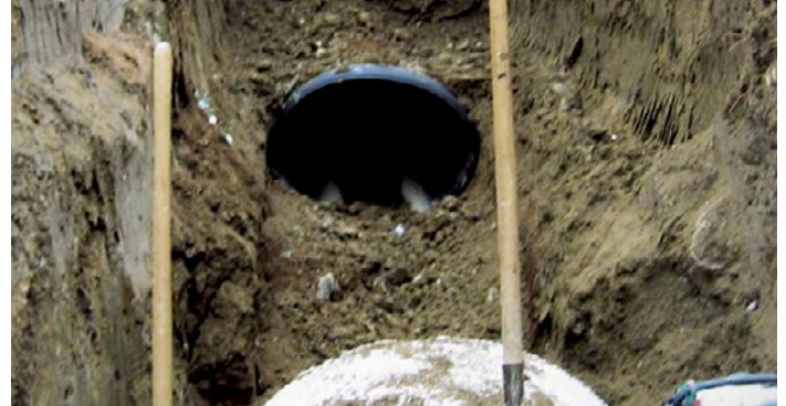
RCP being installed as HDPE is removed
