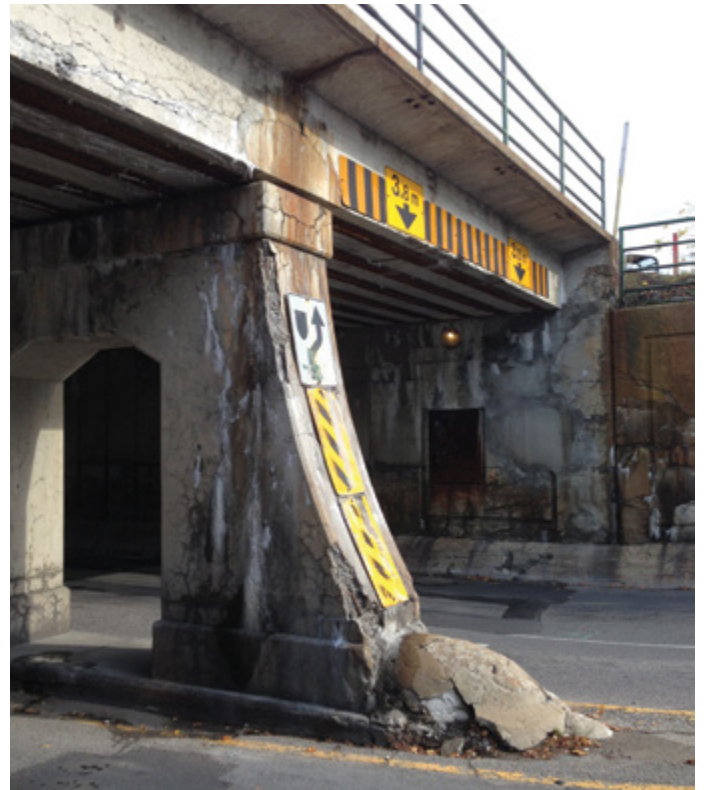
CPR Subway – low ranking bridge condition index Photo courtesy of the CBC
