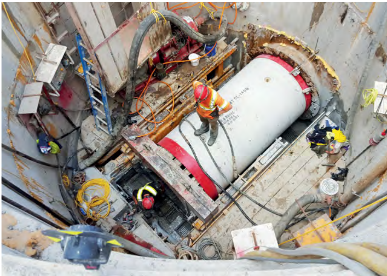
DECAST Concrete Pipe Ready for Installation
