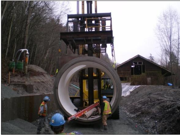
To meet tough design requirements, a higher than normal concrete strength, higher tensile strength of the reinforcing steel, and strict attention to quality assurance was paid to the entire production process. The contractor used the bedding surface for an access road, saving the cost of a temporary road for supplying pipe and equipment.
