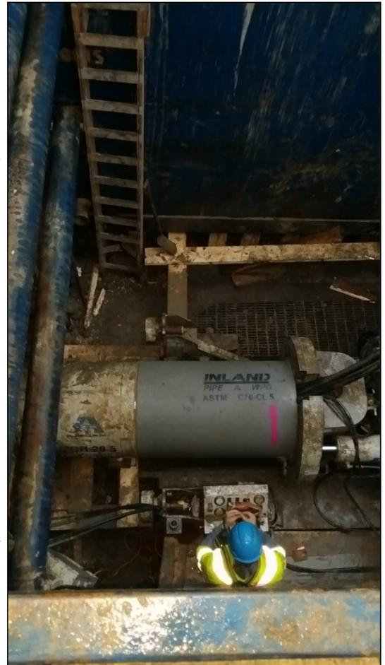
As the excavation moves forward, concrete pipe is jacked behind the cutting face of the auger until it reaches the reception shaft.
