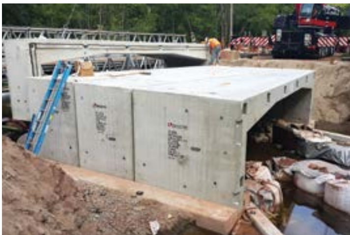
Three-sided precast box units being installed
