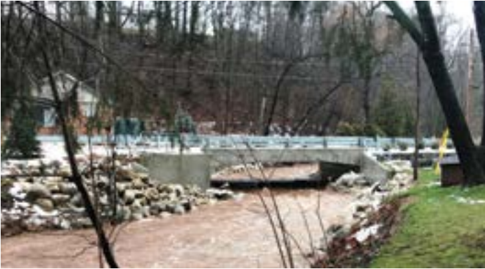
Completed Bridge in Service
