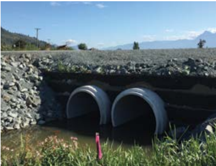
Concrete pipe, with a service life of more than 100 years, is now used for Chilliwack's critical infrastructure
